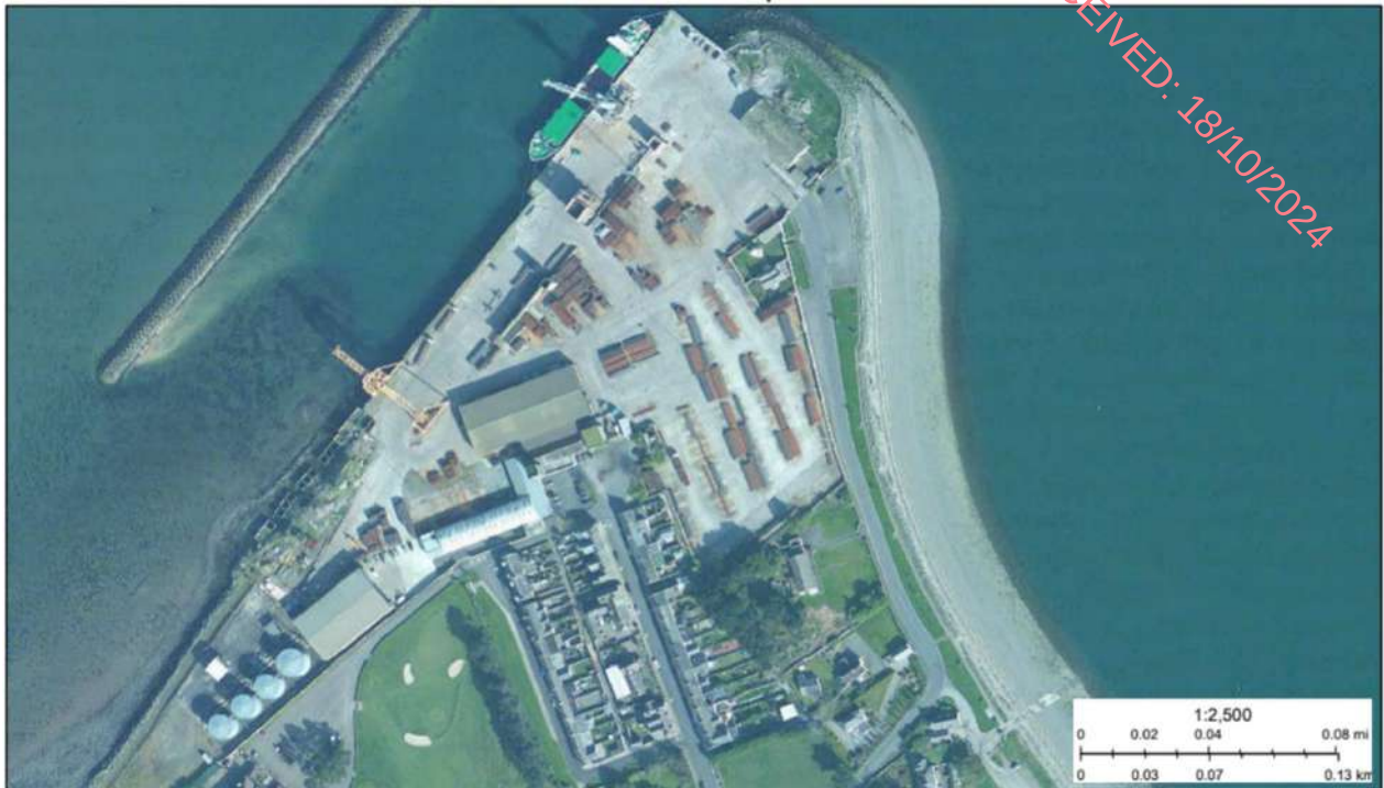
Figure 2-10 OSi Aerial image from 2013 (OSi, 2023)
